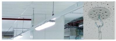
Here a DHI Insulation fixing is used for mounting suspended luminaires in a parking lot. A clean and efficient way of installation.
